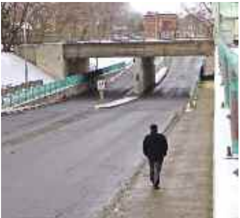
As seen here on February 11, the Westminster underpass will get a facelift this summer. completely re-poured with concrete. The railings, which have rusted over time, are going to be replaced and the retaining walls will be redone. On the west side, the concrete blocks will be removed and the earth will be regraded properly. On the east side, the surface of the concrete wall is going
